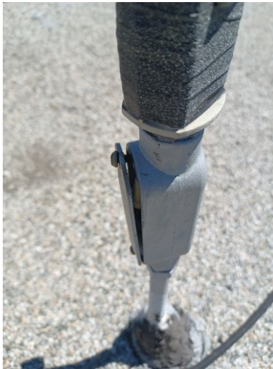
Open conduit on the roof.
